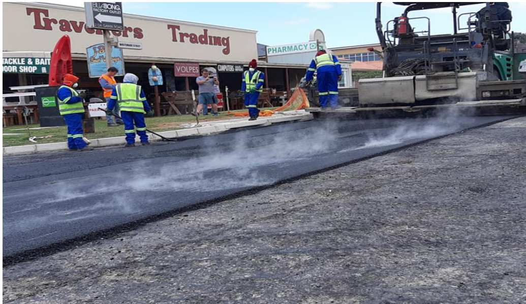
Figure 3: Road building from plastic – Jeffreys Bay, Eastern Cape
